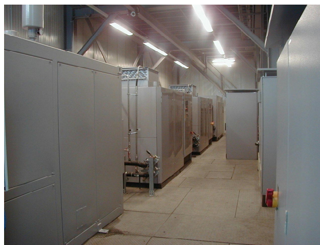
Fig. 2: Compressed air system
