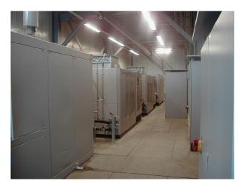
Fig. 2: Compressed air system
